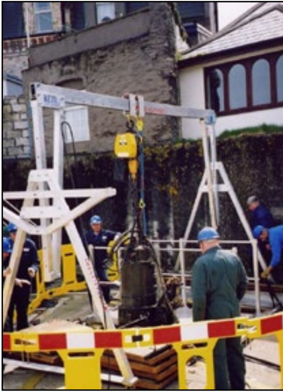
South West Water: Pump maintenance – rapid deployment PORTA-GANTRY WLL 2,000kg with custom “Man-ride restraint” system.
